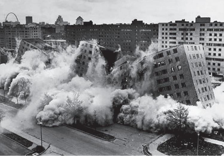
Demolition of Pruitt-Igoe (1972).
